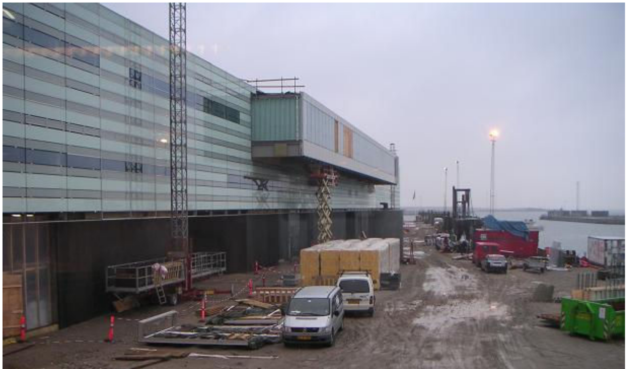
Figure 9: The view from NCC's office on the construction site
